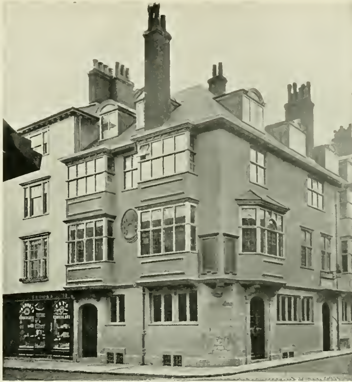
EAST GATE HOTEL, OXFORD. THE MATERIALS ARE FINE ROUGHCAST WASHED WITH COLOUR, HAMMER-DRESSED STONE FROM BRIDGE NORTON, AND SEA-GREEN SLATES. THE SIGN PANEL OF COLOURED CEMENT WAS MODELLED BY GEORGE SYMONDS
